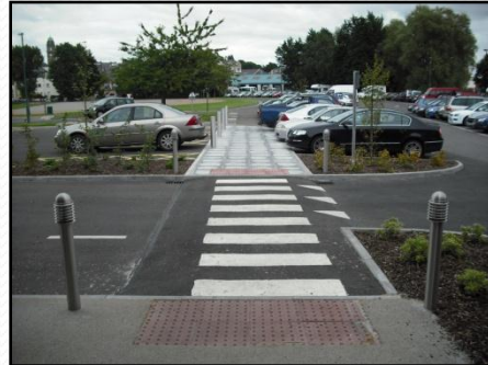
Pathways with tactile paving
