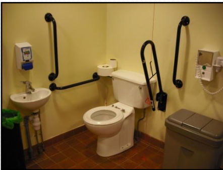
Accessible WC facilities
